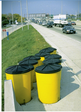
These crash barrels safely remove a car's energy of motion.
